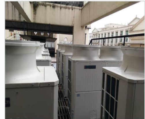
Mitsubishi VRF Condensing Units In a comfort air conditioning project
